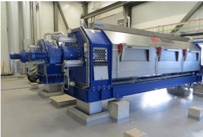
Ekebyverket, Eskilstuna, Sweden - 2 pcs SP-HF09XL screw press and ARU acid rinse equipment
